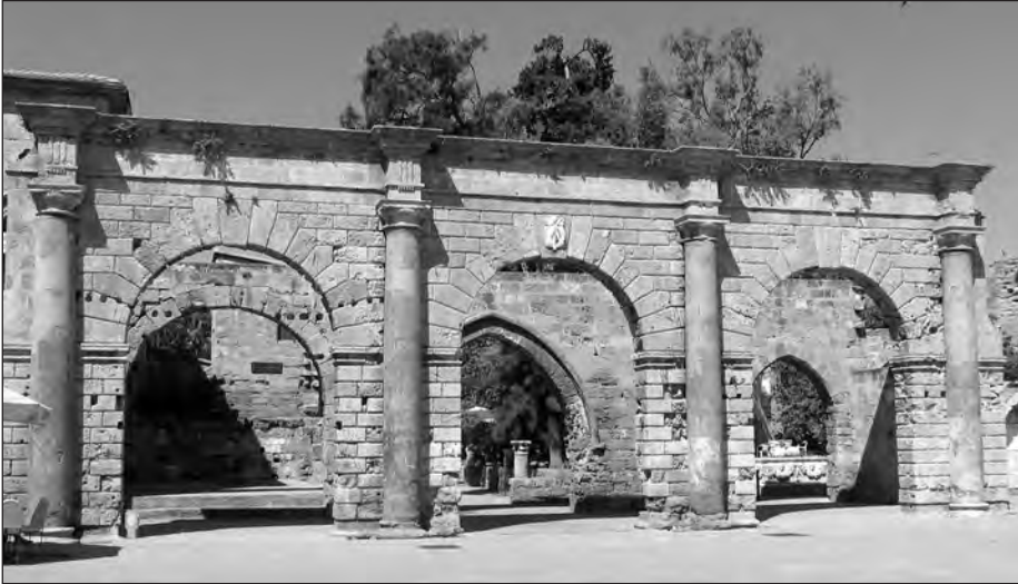
Figure 1. The Triple-arched Gateway of the Palazzo del Proveditore, Famagusta, with Four Granite Spolia Columns from the Greco-Roman City of Salamis – Allan Langdale
